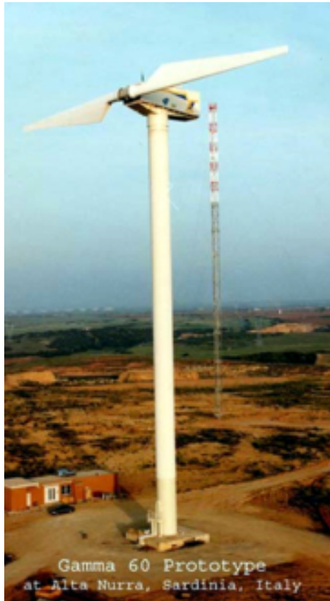
Gamma 60 , the world's first full variable speed wind turbine, 1991, proof of the Seawind concept of yaw control with teetering hinge
